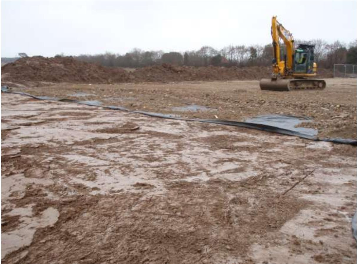
Plate 5. Compound being stripped and covered with Type 2 hardcore
